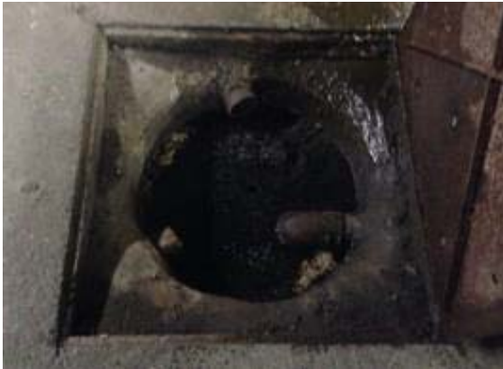
11. Sump Drain A on the west side of the building. We suggest scoping the associated drain pipes to verify their condition.
