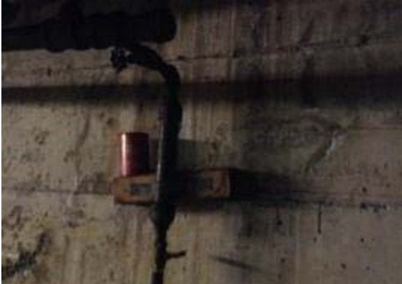
19.Item C stall #14 Water seeping up through crack. A 1ft crack is also apparent behind the wood frame supporting the piping adjacent to the wall.
