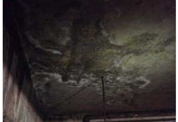
20.Item C stall #14 Water seeping down through ceiling crack. A 10ft crack expanding in diagonal from the West wall of the stall to the Northern Wall and a few branching cracks.
