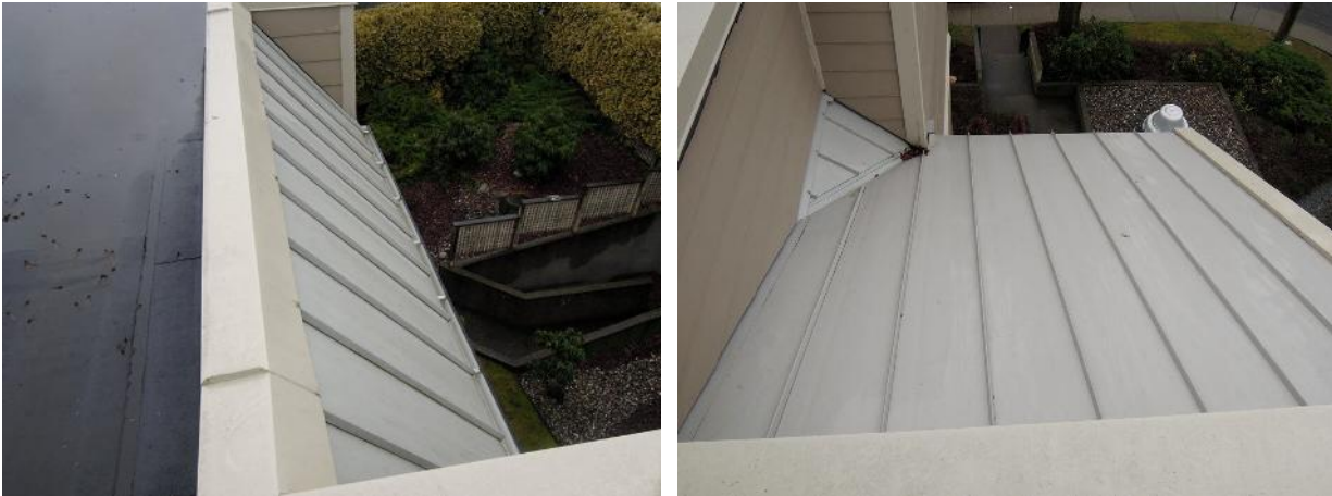
Fig 55. The metal panels extend from the edge of the flat roof (left). A metal panel sloped roof over the west stairwell at Building A (right).
