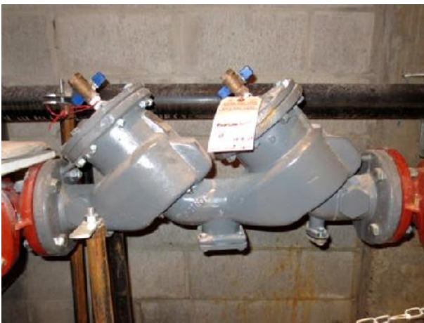
Fig 41. One of the backflow preventers (left). A domestic hot water boiler (right).
