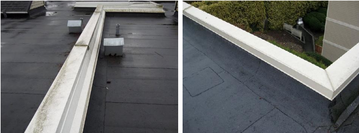
Fig 51. A firewall runs north and south at the midpoint of each building (left). Cap flashings on the parapet walls (right).
