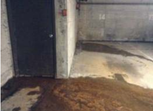
1. Item A.Drainage Problem in Parkade Stairwell. Water pooling in stairwell landing behind door.
