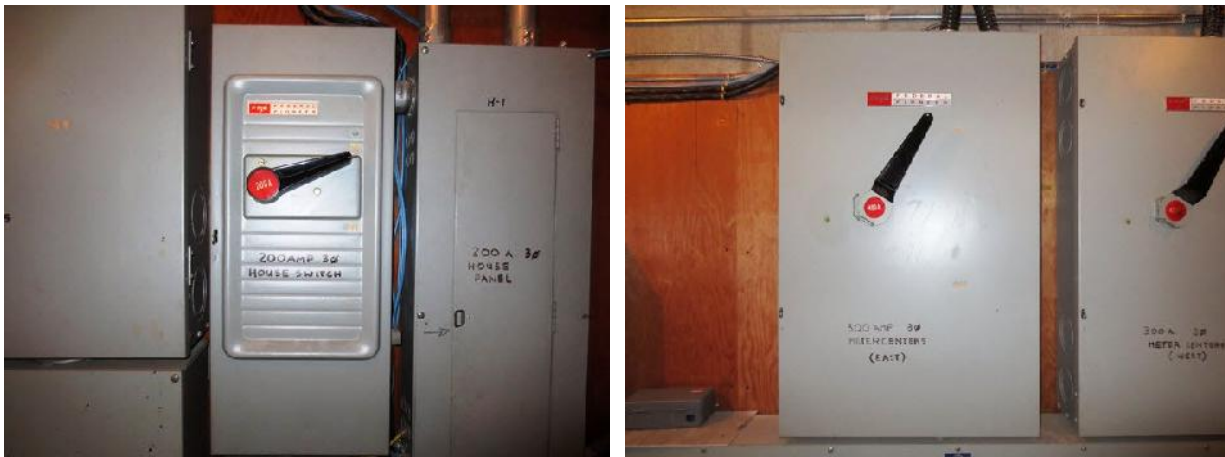
Fig 18. A 200 amp house disconnect (left). A 400 amp unit meter stack disconnect (right).
