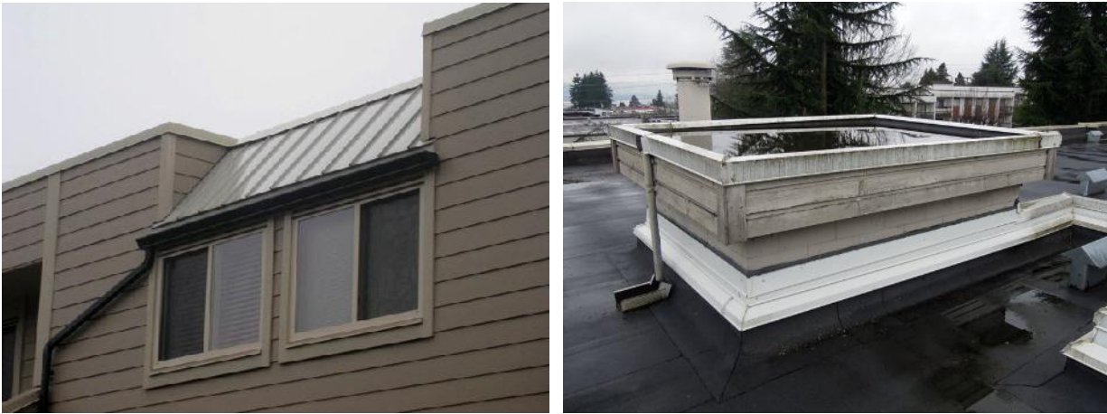
Fig 53. Gutters under a metal panel sloped roof (left). An elevator penthouse (right).
