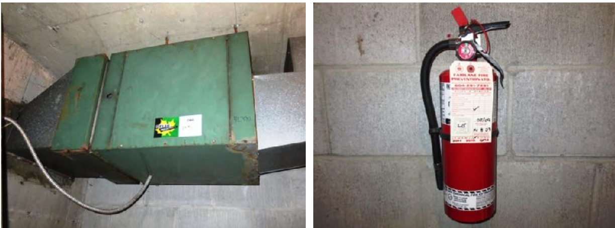
Fig 45. The Delhi inline exhaust fan (left). One of the fire extinguishers (right).
