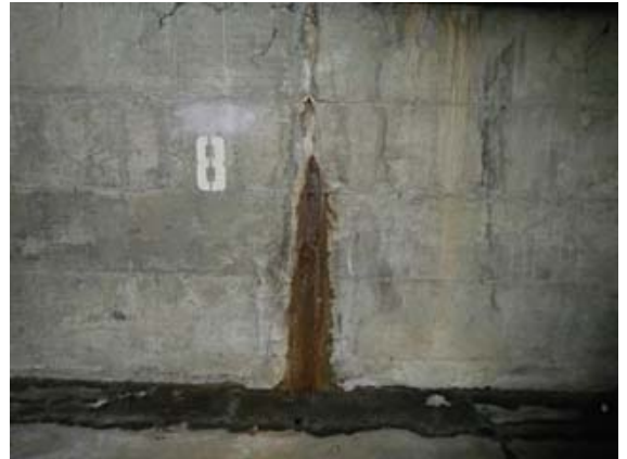
16.Item C stall #8 Water seeping up through cold joint crack and concrete tie void in wall.
