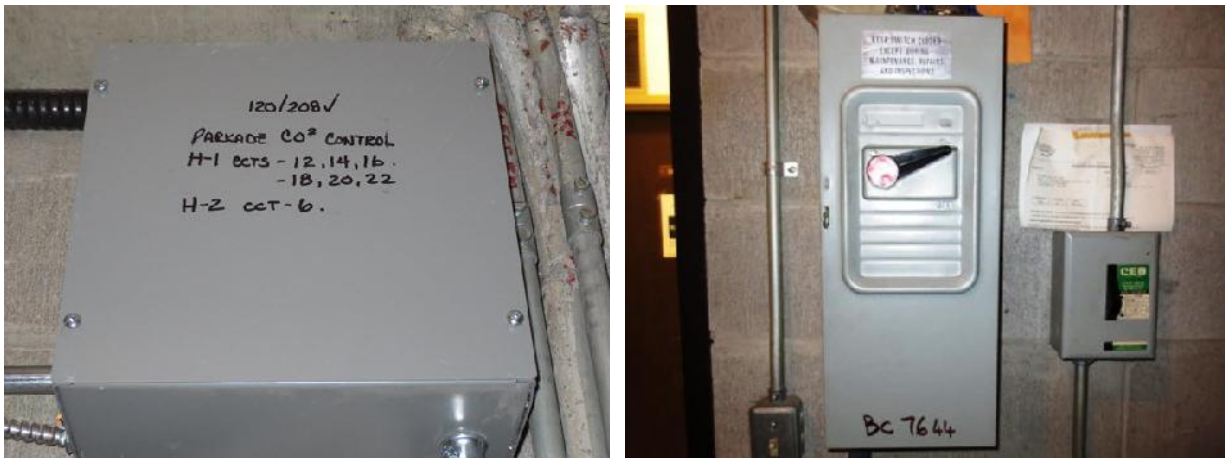
Fig 17. A contactor (left). The elevator disconnects (right).
