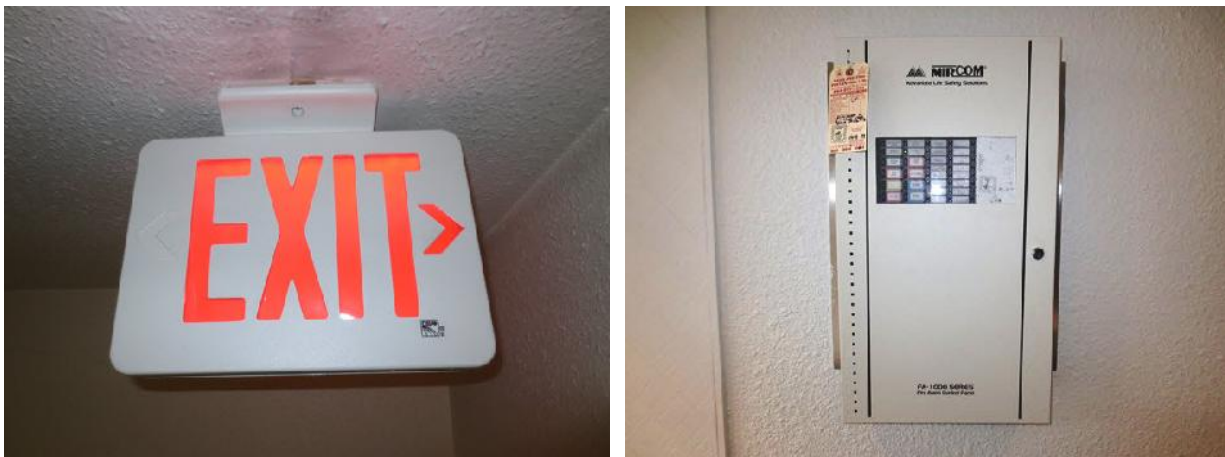
Fig 20. An LED exit sign (left). A fire alarm annunciator panel (right).
