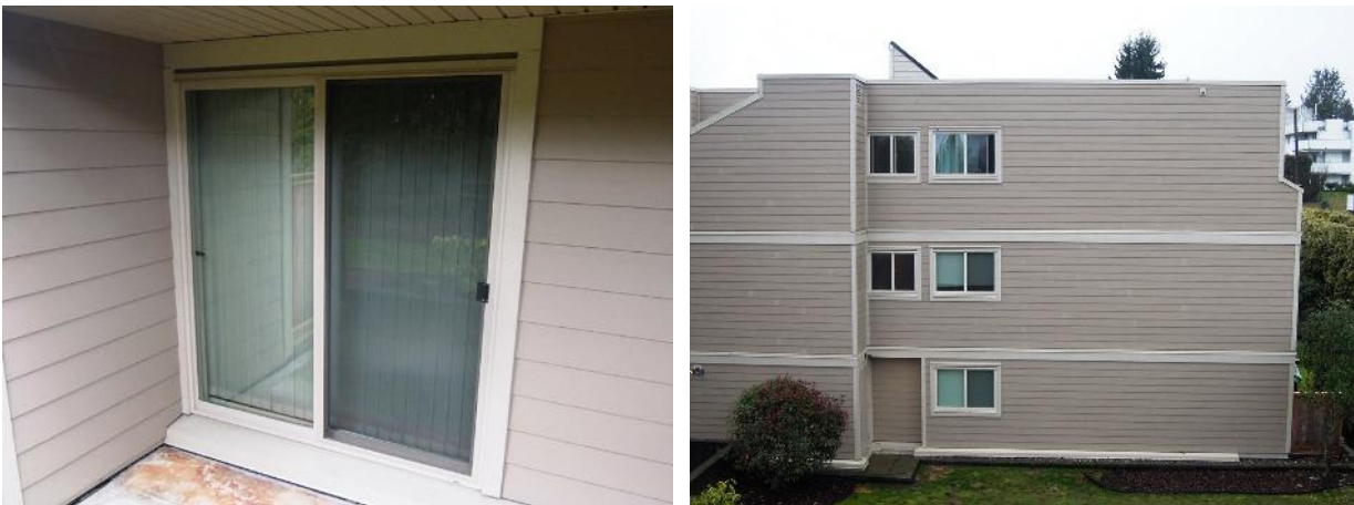
Fig 4. A vinyl double glazed sliding glass door (left). HardiePlank® siding covers the exterior walls (right).
