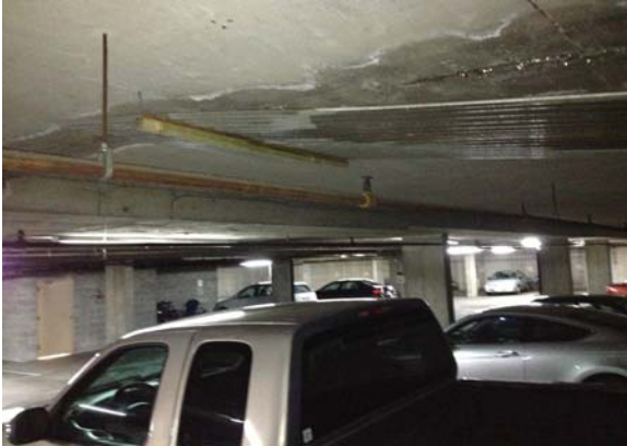
01. Item A Stall # 4-5 15ft ceiling crack emanating from the north wall and ceiling joint expanding outward. We can assume this crack has been leaking for a long period of time as calcite nodules have built up along the
