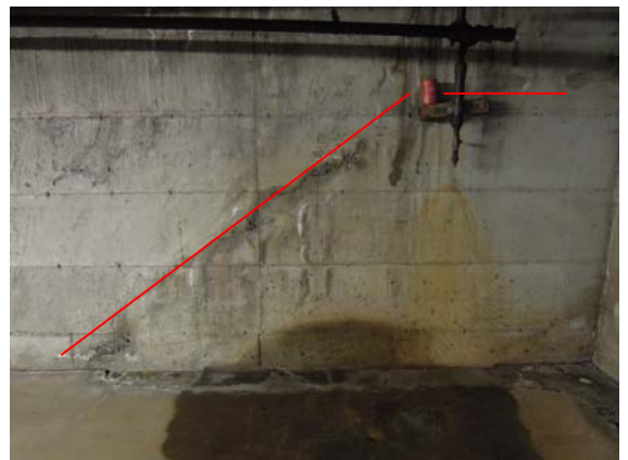
16.Item C stall #8 Water seeping up through cold joint crack and concrete tie void in wall.
