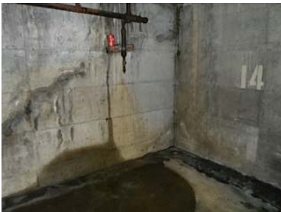
15.Item C stall #7 Water seeping up through cold joint crack void in wall.
