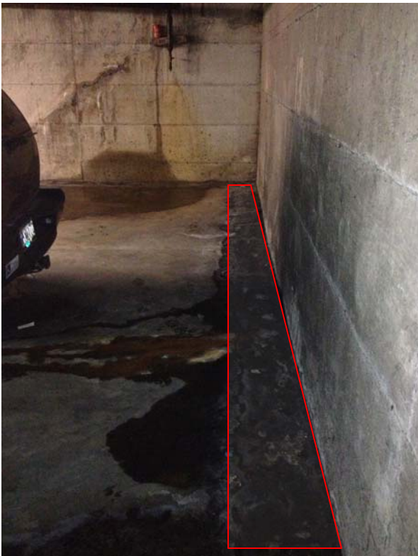
7. Item B. Water ingress along north facing slab to wall interface. Water seeping up through cold joint from below the floor slab. Slight difference in newer concrete installed along wall. Partial length of the wall. Showing the water coming up through the floor.
