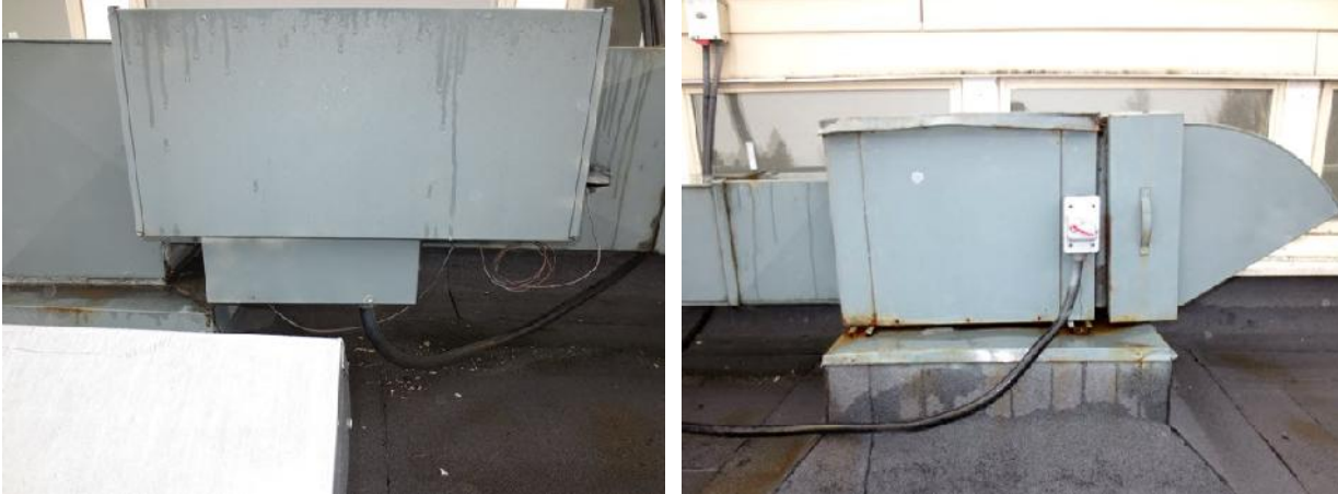
Fig 46. A duct heater (left). One of the make up air units (right).
