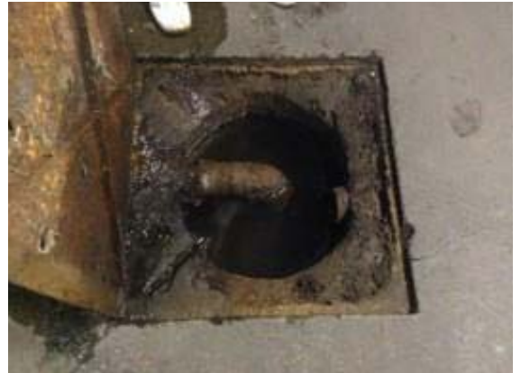
12. Sump Drain B on the east side of the building. We suggest scoping the associated drain pipes to verify their condition.
