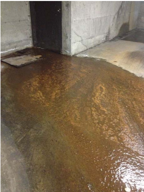
3..Drainage Problem in Parkade Stairwell. Water pooling in stairwell landing behind door and streaming down parkade interior slab to the sump drain.
