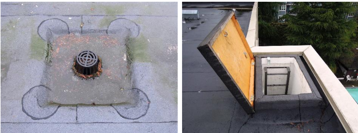
Fig 54. A roof drain (left). A roof hatch and parapet walls (right).
