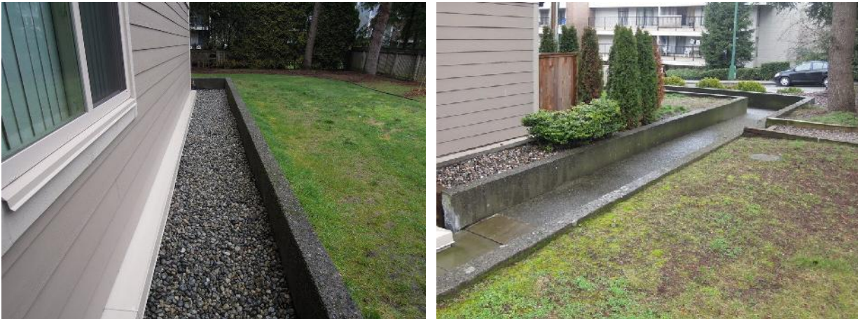
Fig 39. A concrete retaining wall and a drainage corridor (left). Concrete retaining walls at the border of a sidewalk (right).
