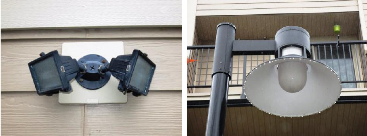
Fig 25. Halogen spot lights at the side of a building (left). A front entrance post lamp (right).
