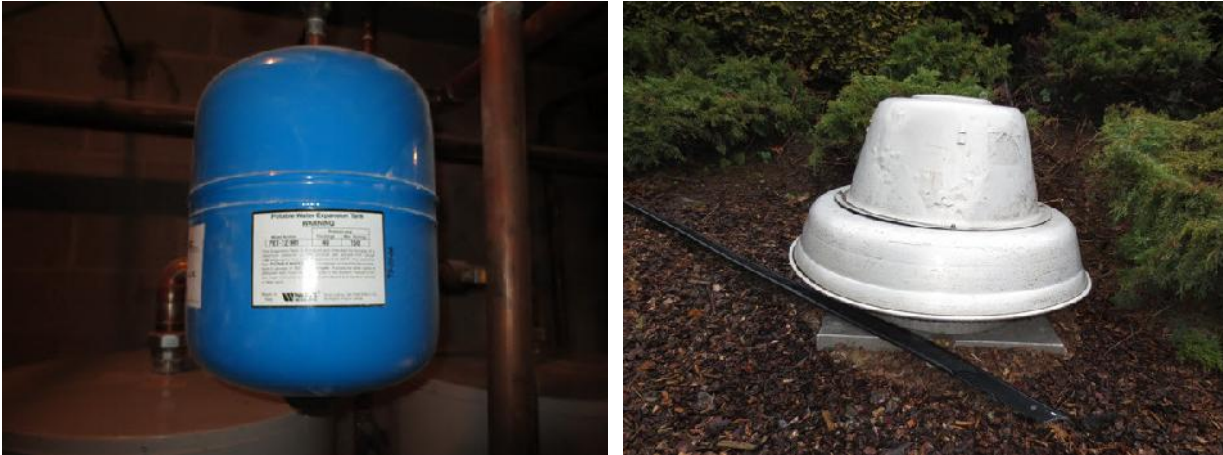
Fig 44. A water pressure expansion tank (left). A domed parkade exhaust fan situated on the grounds (right).
