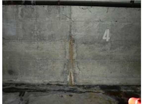
15.Item C stall 4-5. Water seeping up through cold joint void in wall.
