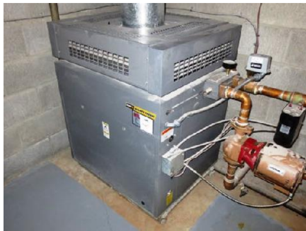
Fig 41. One of the backflow preventers (left). A domestic hot water boiler (right).
