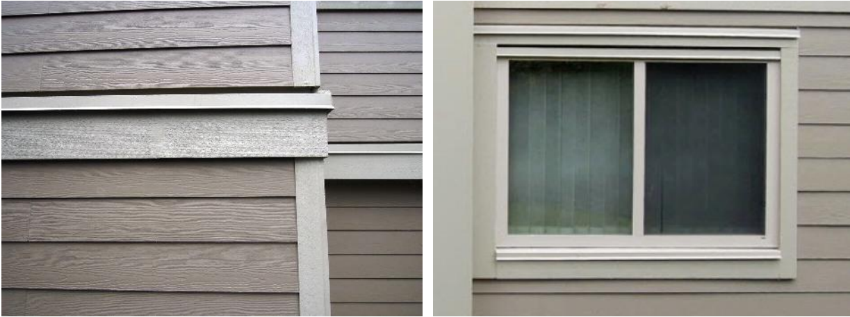
Fig 5. A close up view of the HardiePlank® siding (left). Flashings are visible at the top and bottom of the vinyl windows (right).
