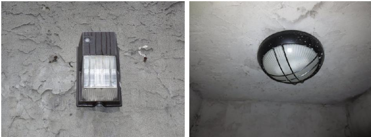
Fig 24. A high bay light over a parkade entrance (left). A marine light in one of the parkade stairwells (right).
