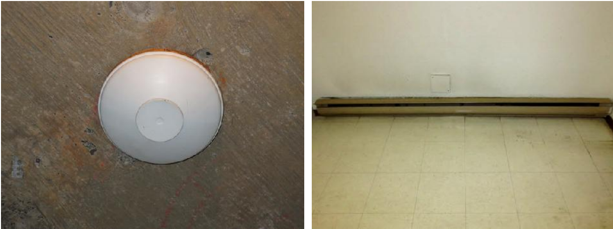
Fig 21. A heat detector (left). An electric baseboard heater in the basement (right).
