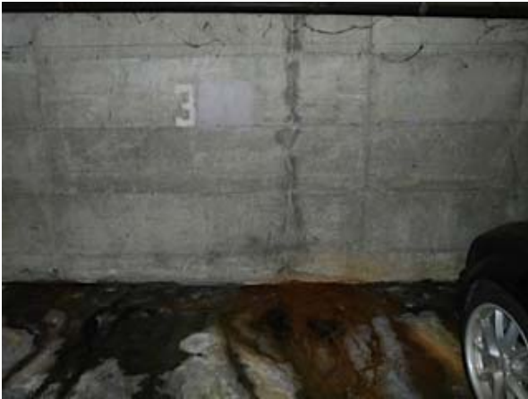
5. Item B. Water ingress along north facing slab to wall interface. Water seeping up through cold joint from below the floor slab.
