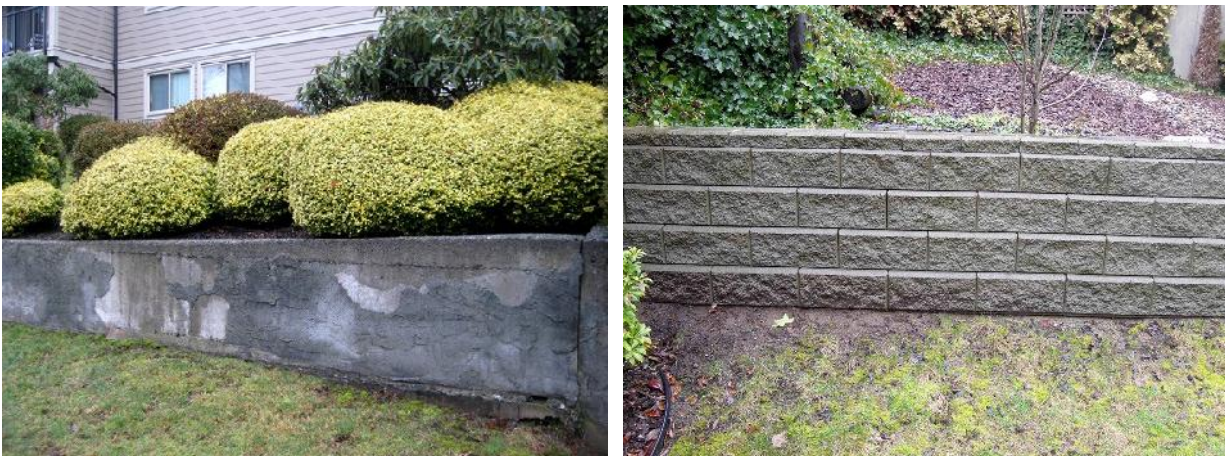
Fig 40. A concrete retaining wall at the front of the property (left). The Allen block retaining wall behind Building B (right).
