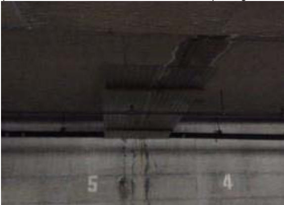
03. Item A Stall # 4-5 15ft ceiling crack emanating from the north wall and ceiling joint expanding outward.
