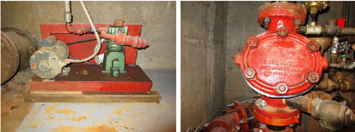
Fig 49. The compressor in the mechanical room at Building A (left). One of the dry pipe valves (right).
