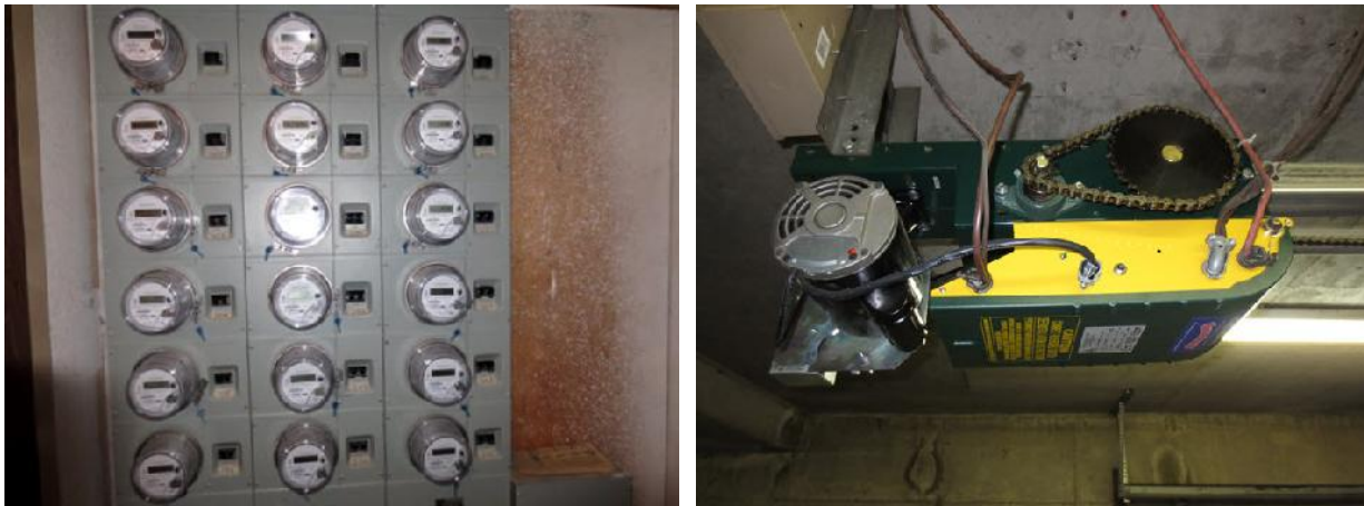
Fig 28. A set of unit meter stacks (left). The new overhead door opener in Building A (right).
