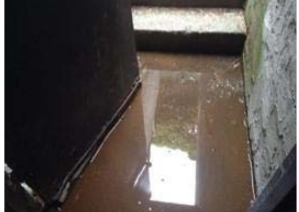
2..Drainage Problem in Parkade Stairwell. Water pooling in stairwell landing is saturated with soil.
