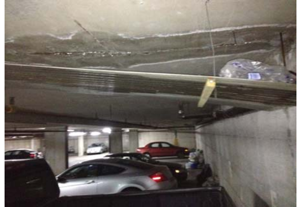
02. Item A stall # 4-5 01. Stall # 4-5 15ft ceiling crack a corrugated panel has been installed below the leaking area of the crack to divert the leaking water away from the parking stall.
