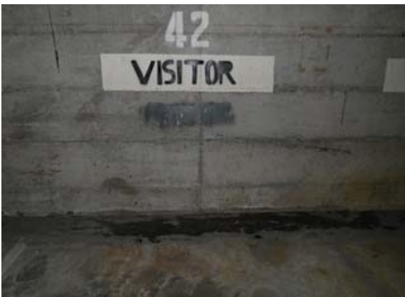
23.Item C-1 stall #42 Additional non active cracks.
