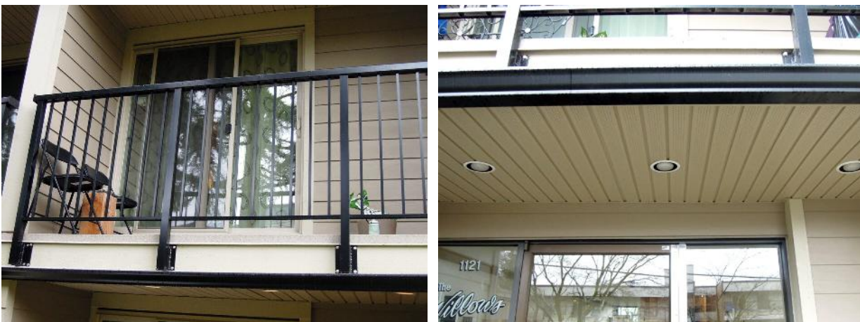
Fig 7. Balcony railings are black metal (left). A view of the vinyl soffits over a building front entrance (right).
