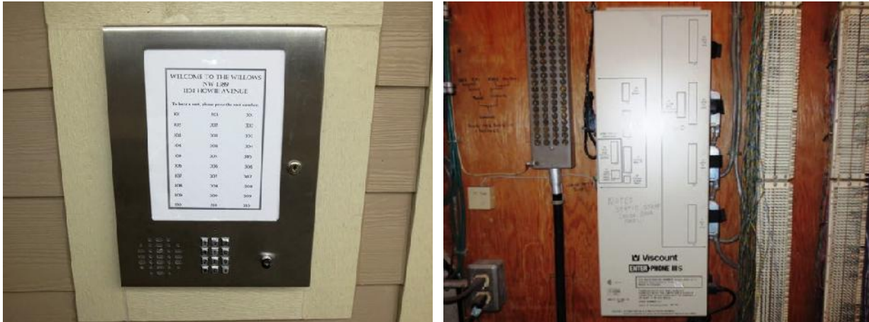
Fig 19. The enterphones are outside the main entrance (left). An enterphone control relay (right).
