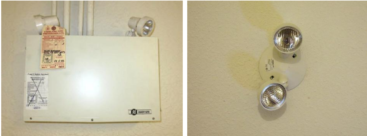
Fig 23. A dual head emergency light battery backup (left). A dual remote head (right).
