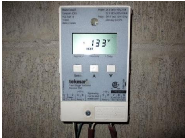
Fig 42. A carbon monoxide sensor (left). An electronic boiler controller (right).
