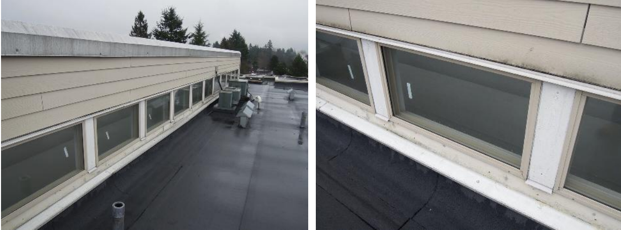
Fig 57. The windows in the vaulted roofs on Building A are double glazed with vinyl frames.
