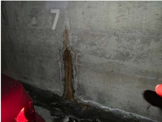
15.Item C stall #7 Water seeping up through cold joint crack void in wall.
