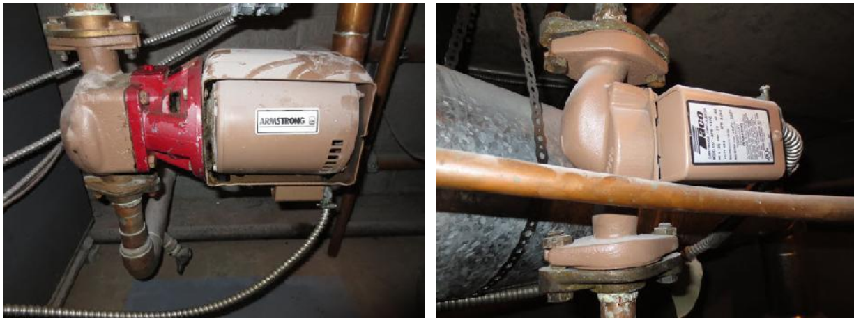
Fig 48. A circulation pump (left). A recirculation pump (right).
