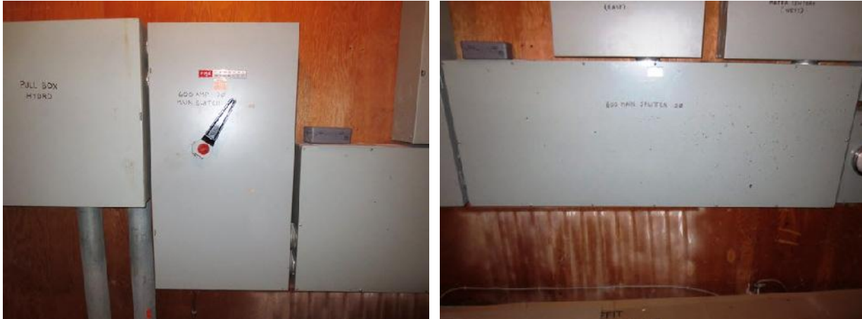
Fig 27. One of the main building disconnects (left). A main splitter (right).
