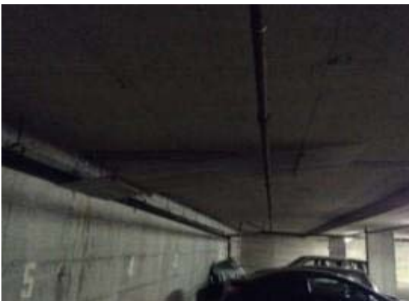
05. Item A Stall # 4-5 15ft ceiling crack emanating from the north wall and ceiling joint expanding outward.
