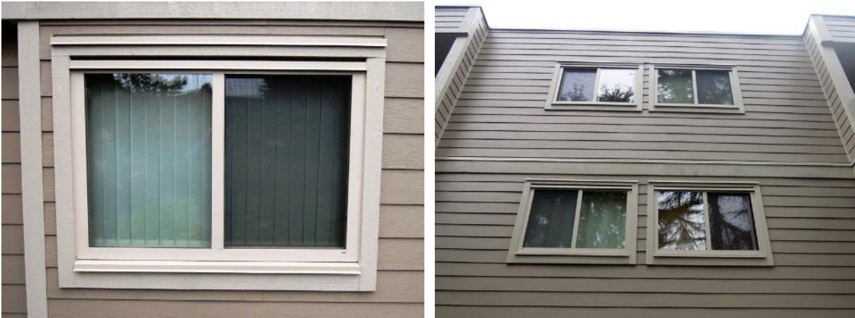
Fig 8. Painted fir/hem trim boards are around the windows (left). A view of upper floor windows (right).
