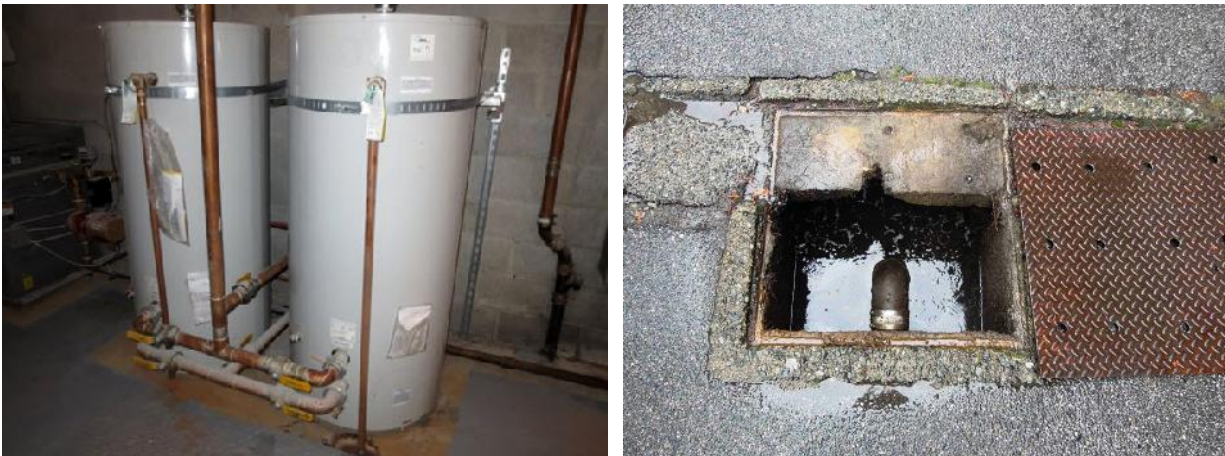
Fig 50. A set of hot water storage tanks (left). This gravity sump is on one of the entrance ramps (right).
