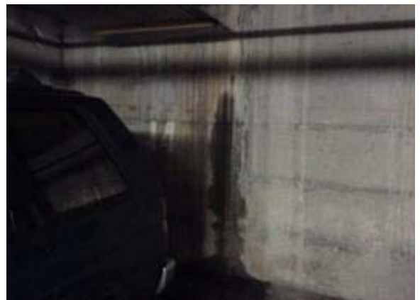
06. Item A Stall # 14 (Active) 5 lf of wall cracks Crack from base to the upper end of the wall. The crack is actively leaking from the mid wall.
