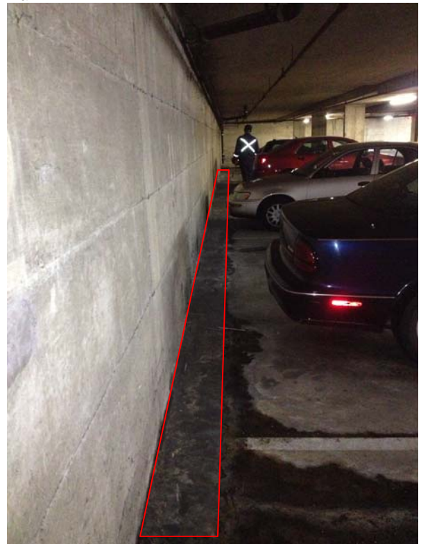
6. Item B. Water ingress along north facing slab to wall interface. Water seeping up through cold joint from below the floor slab. Slight difference in newer concrete installed along wall.
