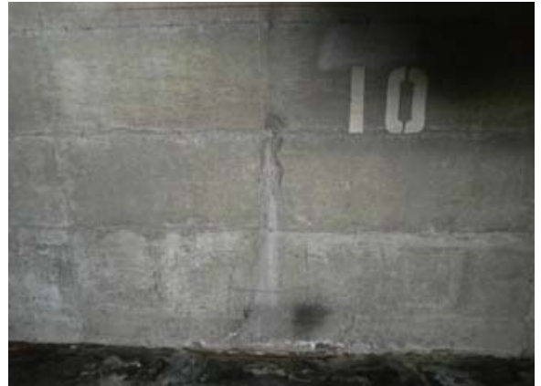
22.Item C-1 stall #10 Additional non active cracks.
