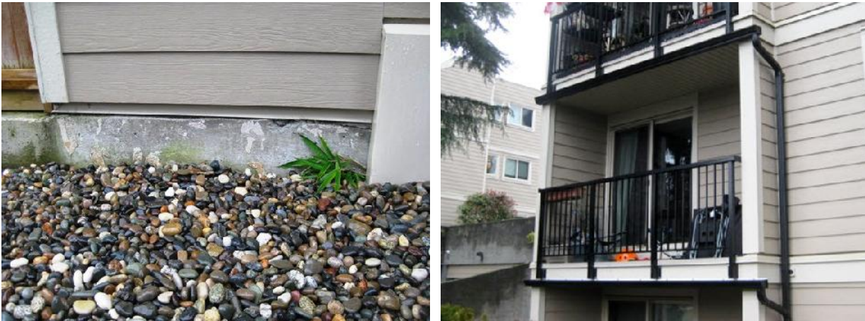
Fig 6. A section of the concrete foundation (left). The gutter system at balconies (right).
