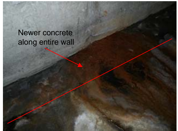
6. Item B. Water ingress along north facing slab to wall interface. Water seeping up through cold joint from below the floor slab. Slight difference in newer concrete installed along wall.
