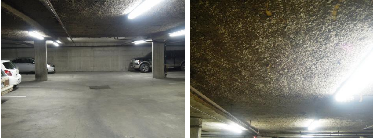
Fig 62. Another view of the slab on grade (left). An insulated section of the suspended slab (right).
