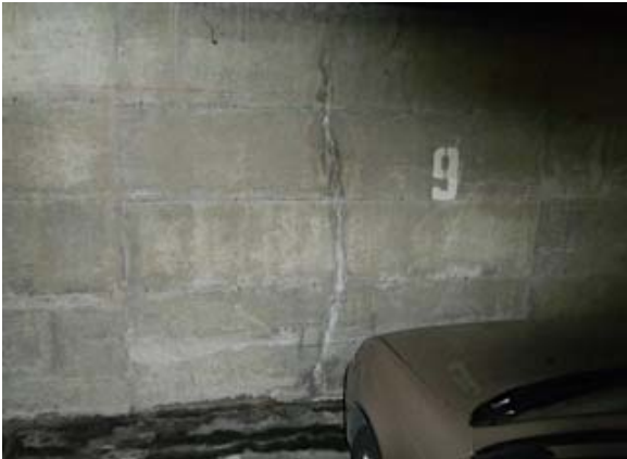
21.Item C-1 stall #9 Additional non active cracks.
