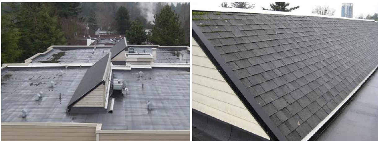
Fig 56. A view of the vaulted roofs on Building B (left). Laminate asphalt shingles on a vaulted roof (right).
