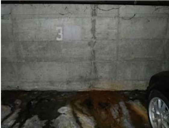
14.Item B. Water ingress along north facing slab to wall interface. Water seeping up through cold joint from below the floor slab.
